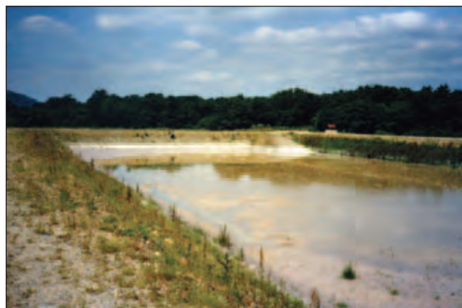
Surface water settlement lagoon to separate solids before discharge to the River Teign.
